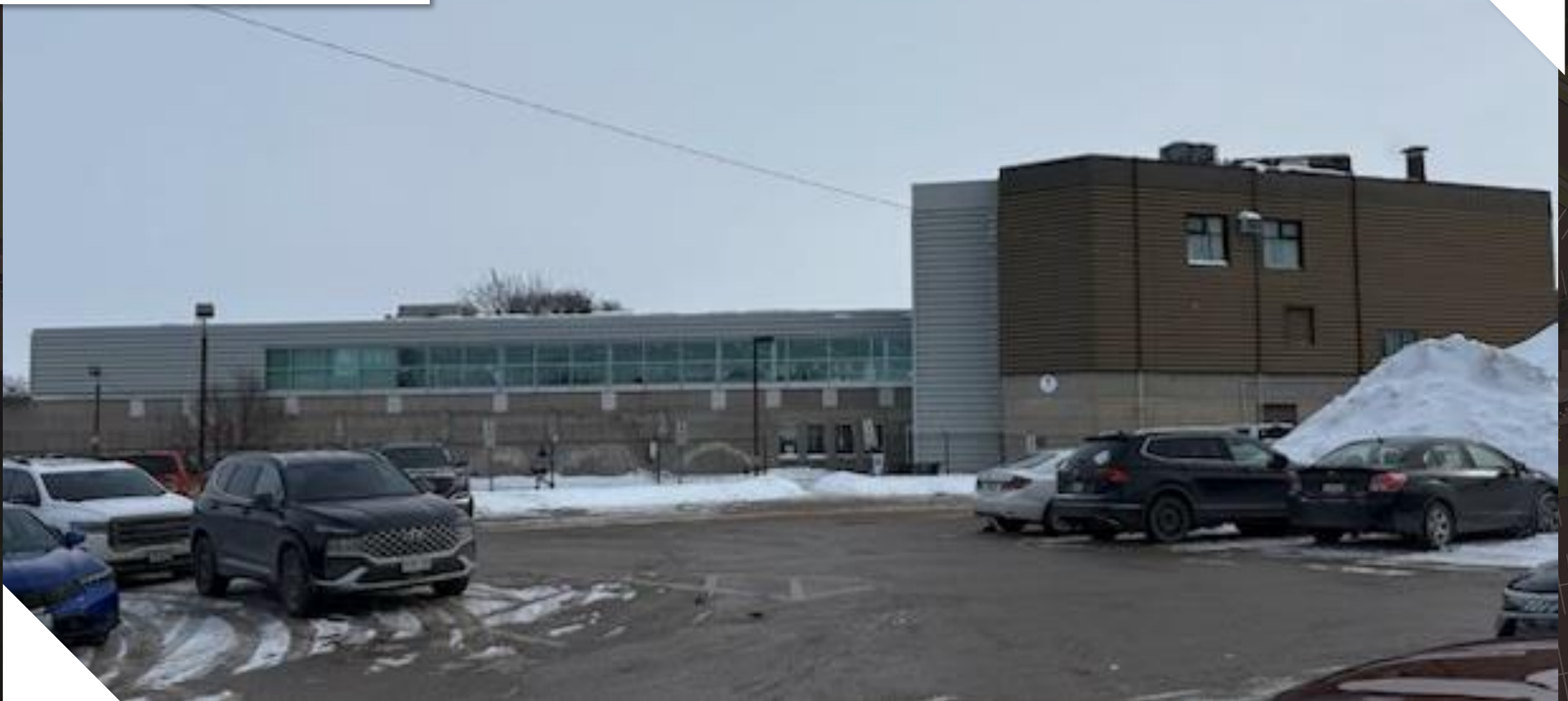
West view of Existing YMCA
