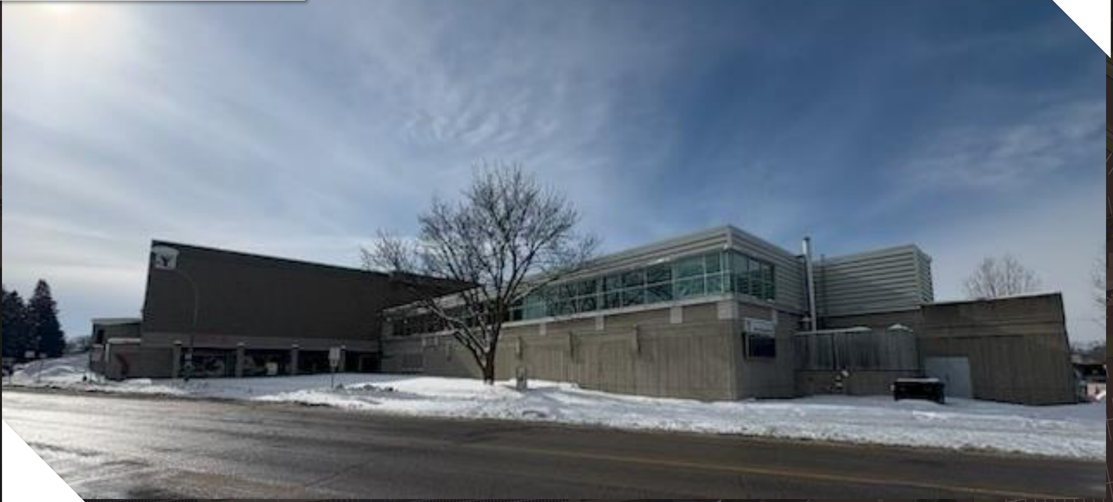
Northwest view of Existing YMCA
