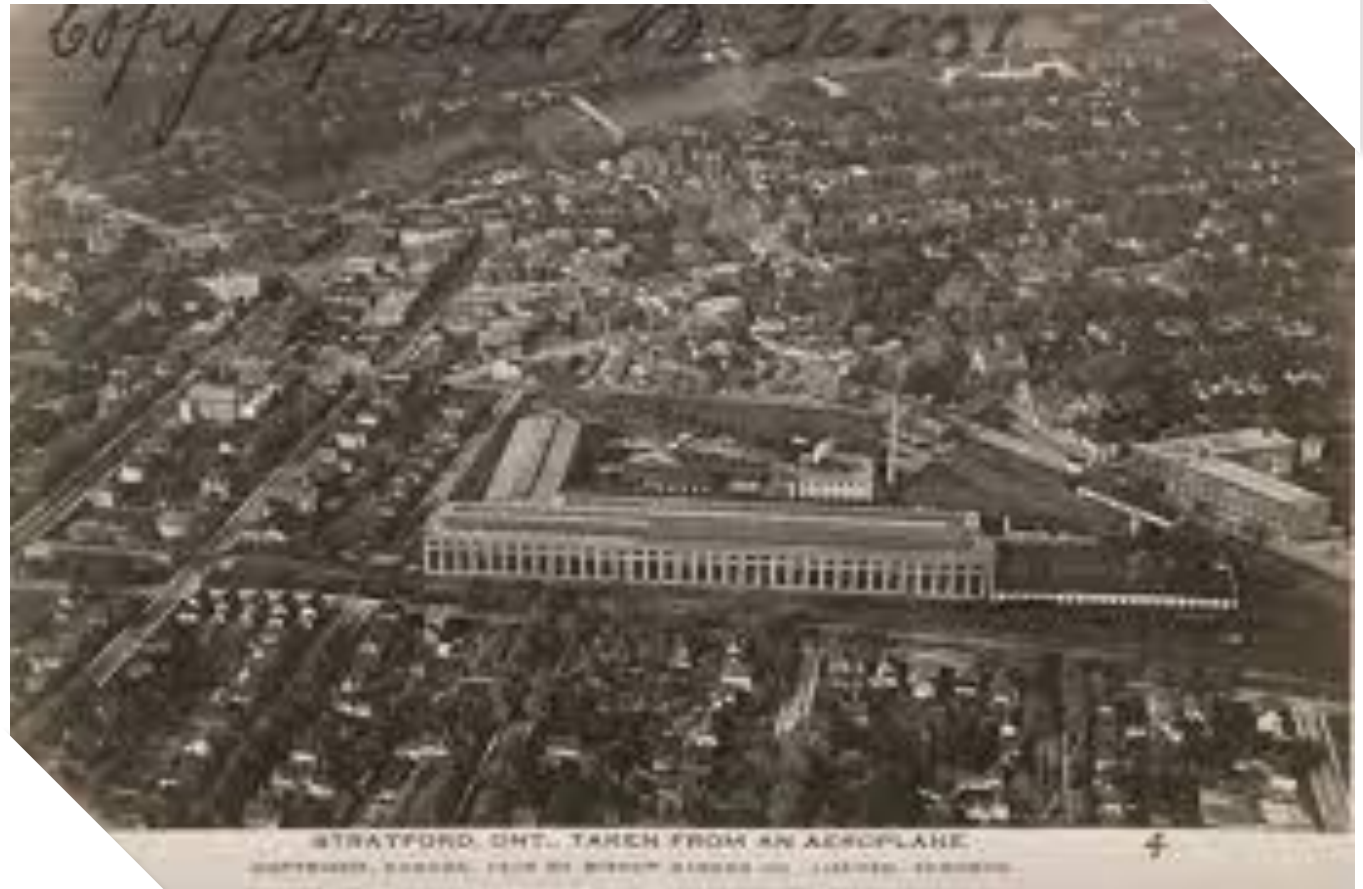
South aerial view of the GTR
